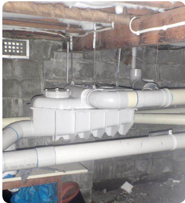
Retrofit installation suspended under the house
