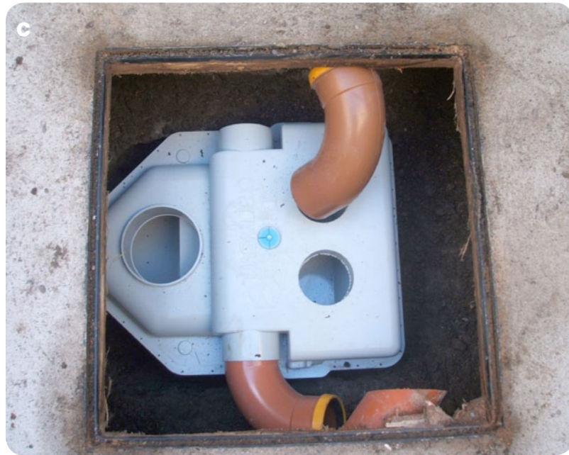
A. Slab on ground with a typical in ground Drainwave installation. B. In ground installation using Kitchen greywater as wash down. C. In ground installation in a manhole which collects water from the roof and patio before releasing to the main sewer. D. Retrofit installation suspended under the house
