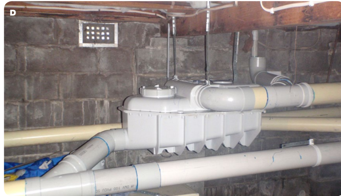
A. Slab on ground with a typical in ground Drainwave installation. B. In ground installation using Kitchen greywater as wash down. C. In ground installation in a manhole which collects water from the roof and patio before releasing to the main sewer. D. Retrofit installation suspended under the house
